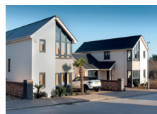
CAVANNA BUILD Primrose Hill, Torquay
